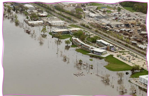
River Drive flooding
