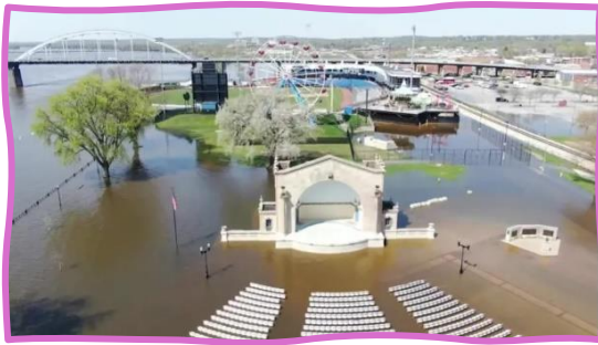
2 Flooding of Ballpark in the QC in 2019
