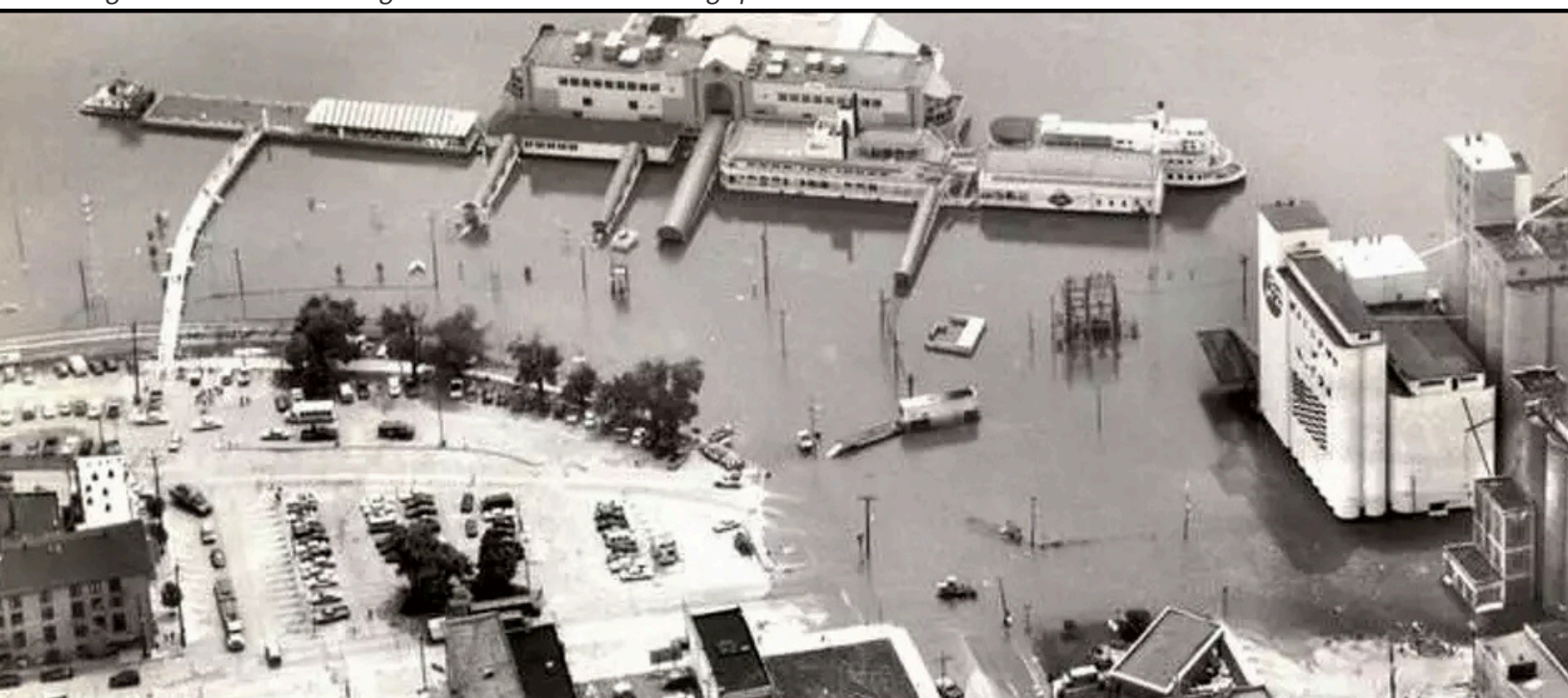
Aerial image of Alton's riverside during summer 1993 / The Alton Telegraph
